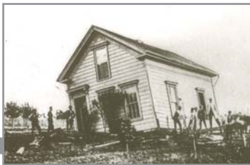
1868—Damage in Hayward
