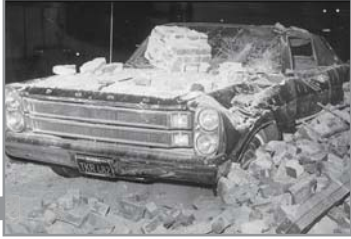
1969—Damage in Santa Rosa
