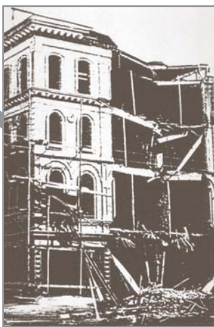
1865—Damage in San Francisco
