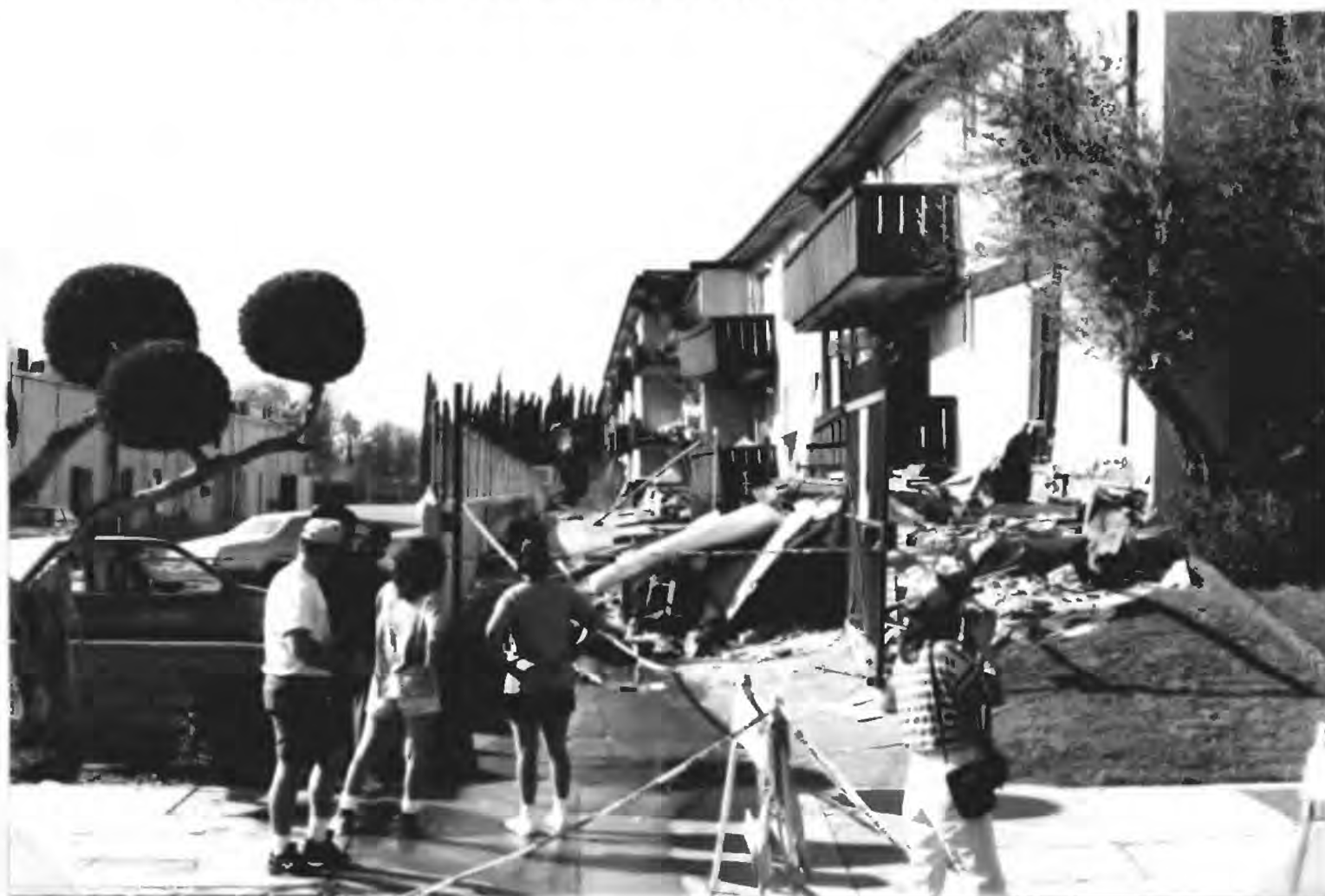
Figure 8. Northridge Meadows apartment complex, Northridge( listed under intensity IX). Collapsed building in right foreground was formerly at same height as, and aligned with, uncollapsed building in middle background.
