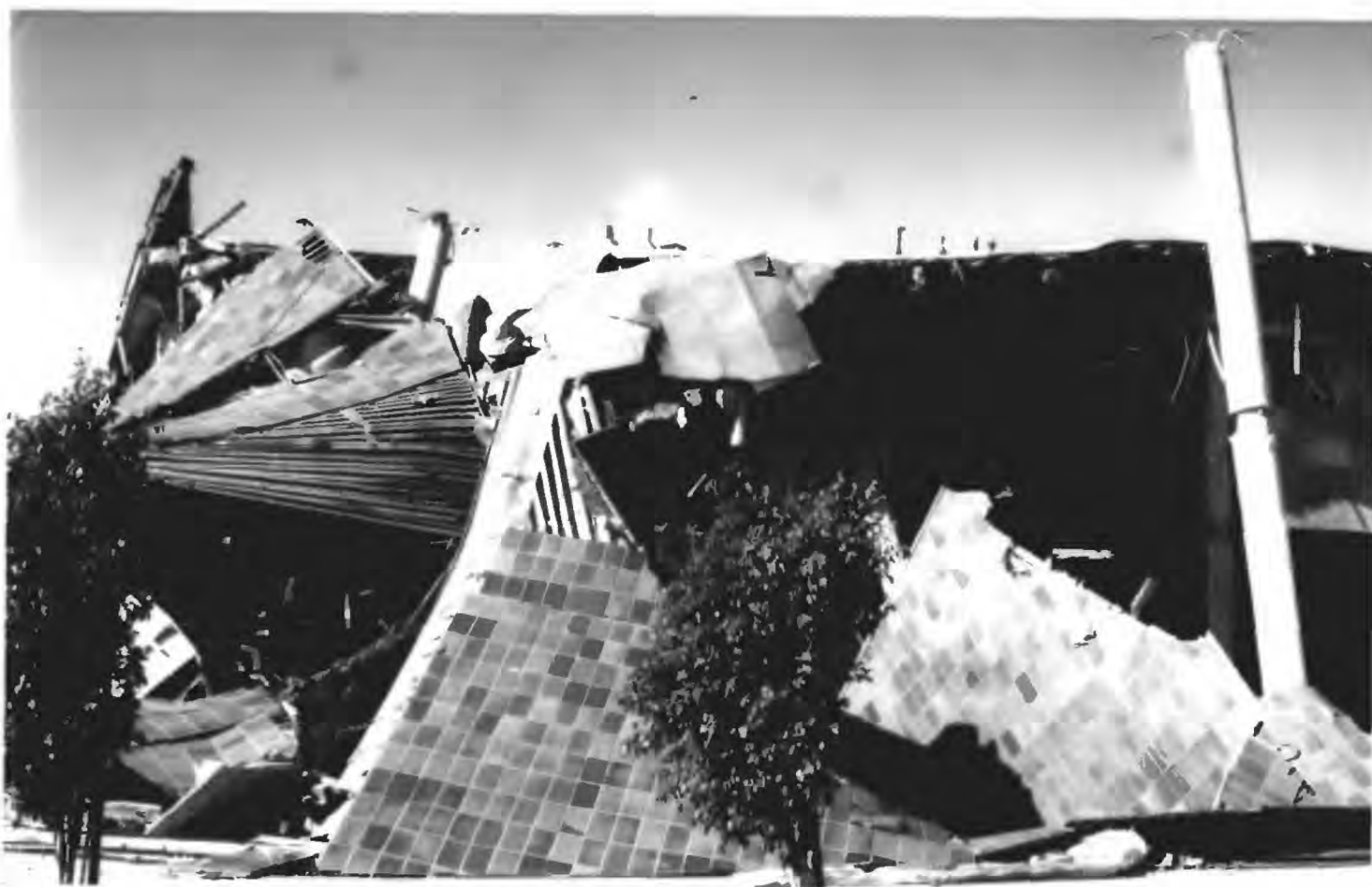
Figure 6. Collapse of Bullocks department store at the Northridge Fashion Mall, Northridge (listed under intensity IX). The notch on the standing column shows where a floor slab had been attached.
