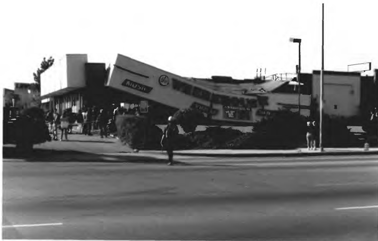
Figure 7. Partial collapse of a store building in a shopping center near the Northridge Fashion Mall, (listed under intensity IX).
