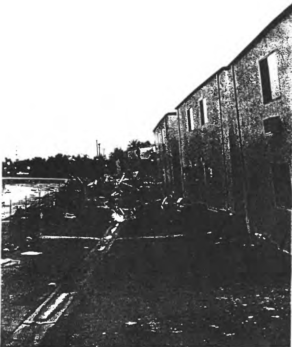
Figure 19. Collapse of apartment buildings onto underlying parking areas, Reseda (listed under intensity VIII). Debris in middle background resulted from fighting a fire in the destroyed building that was triggered by an aftershock.
