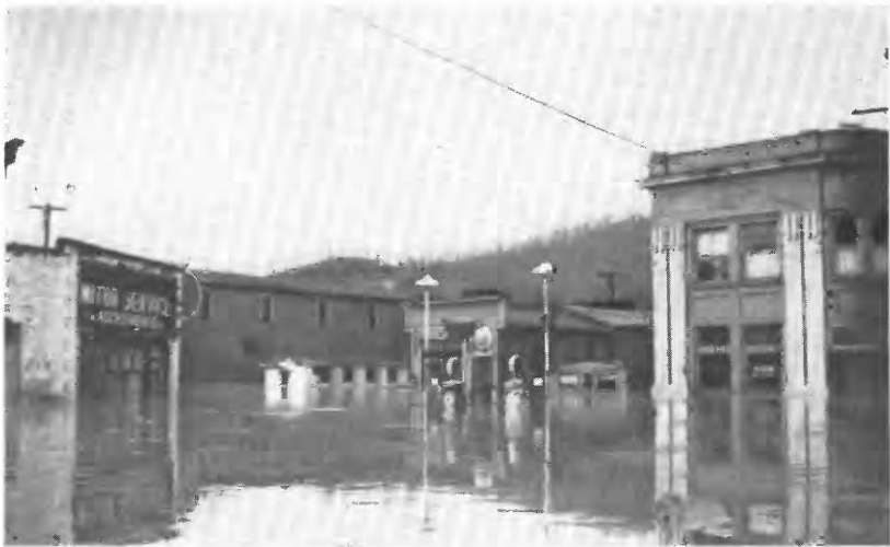
FIGURE 17.—Business section of Burnsville during flood of April 16, 1939. Stage is about 1.5 feet lower than the maximum August 5, 1943. Courtesy of Corps of Engineers.
